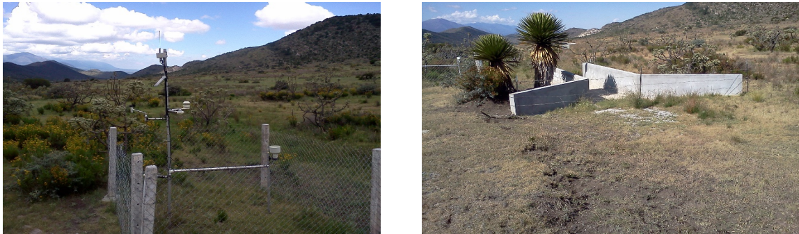
Figure 3. Weather station and gauge canal of surface runoffs at the Experimental Watershed in Saltillo, Coah.
